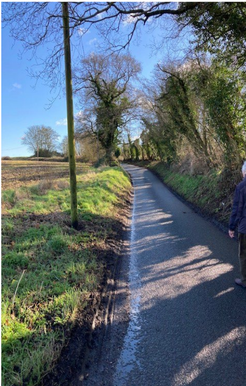
3. Damage to verges and unsighted road
