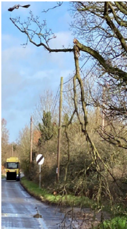
56. Extensive damage already done to low hanging trees – no warning signage
