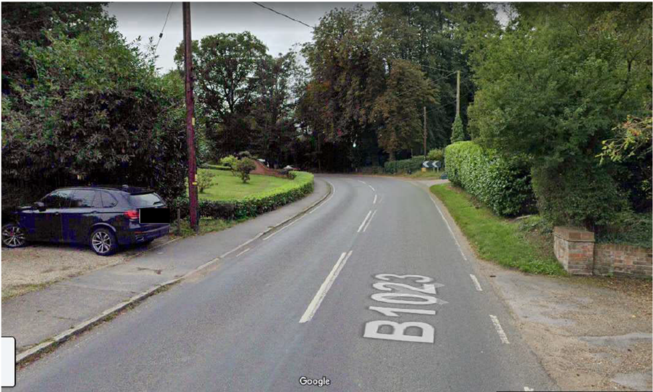
B1023 approaching All Saints Church (looking south) – shows frequency of accesses, narrow verges, low radius (approximately 75m) curve and limited visibility
