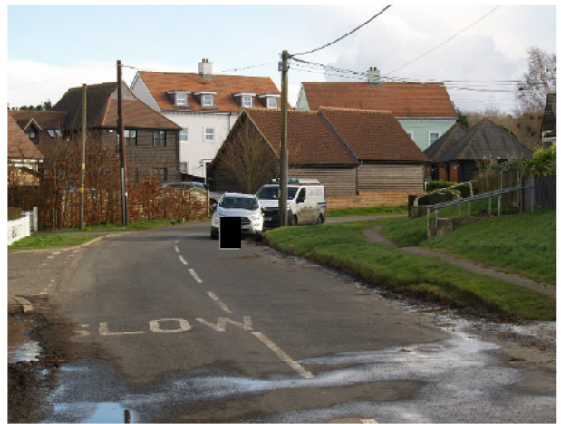
72. School Road showing the short section of footpath around the bend in the road.
