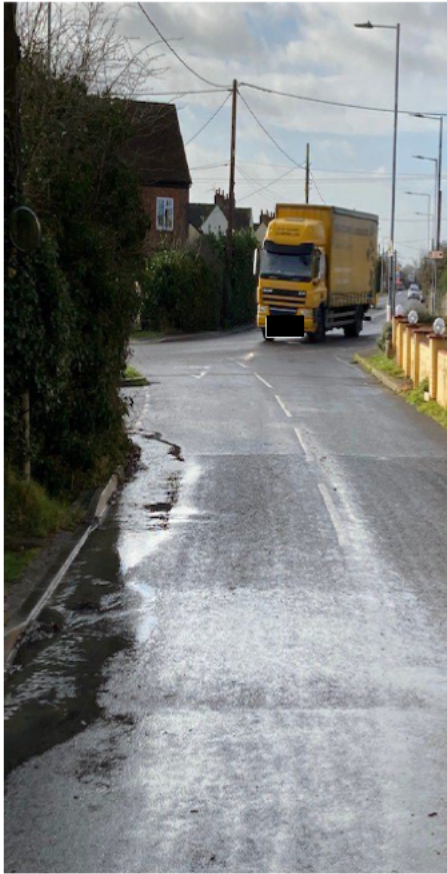
58. Accident black spot for obscured right turn
