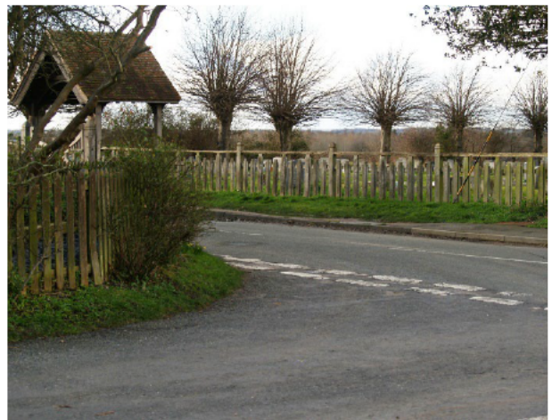
70. Blind Junction with Kelvedon Road
