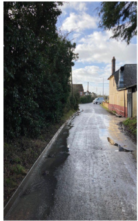
57. Towards B1023 junction showing narrow 2.8m width
