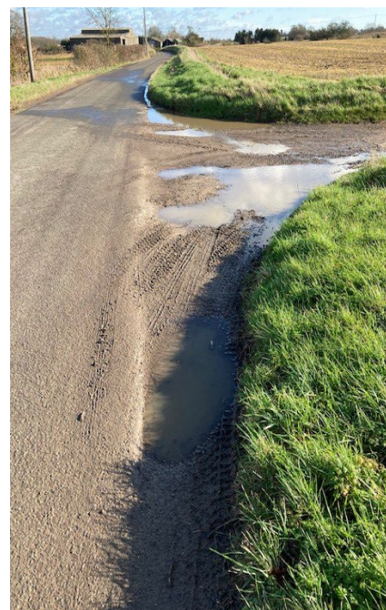
8. Extensive damage to private access as traffic uses this as a passing place
