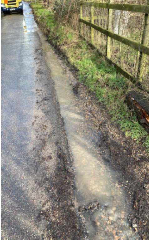
54. To illustrate extensive damage already made as traffic is forced to make passing places
