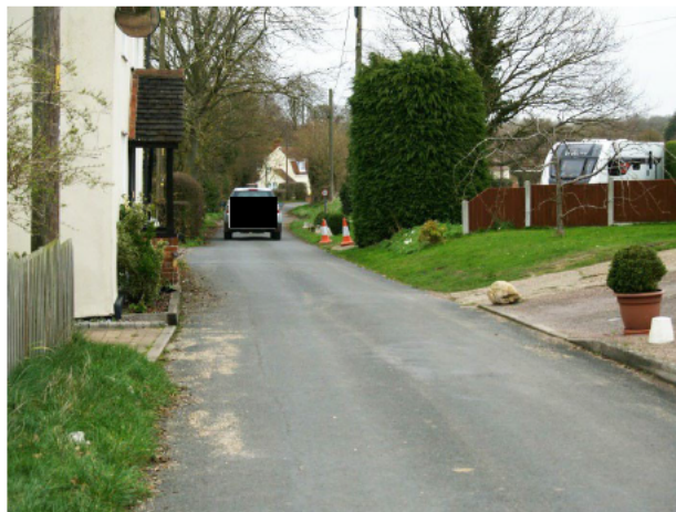
45. Showing the road width from 120m onwards
