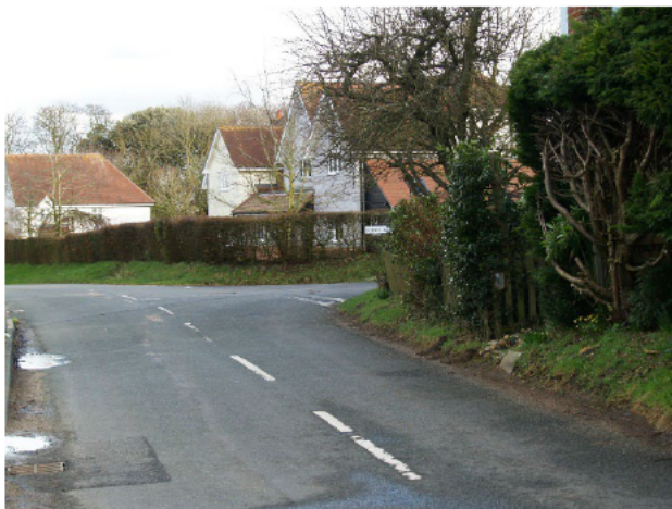
71. View from Kelvedon Road showing blind junction
