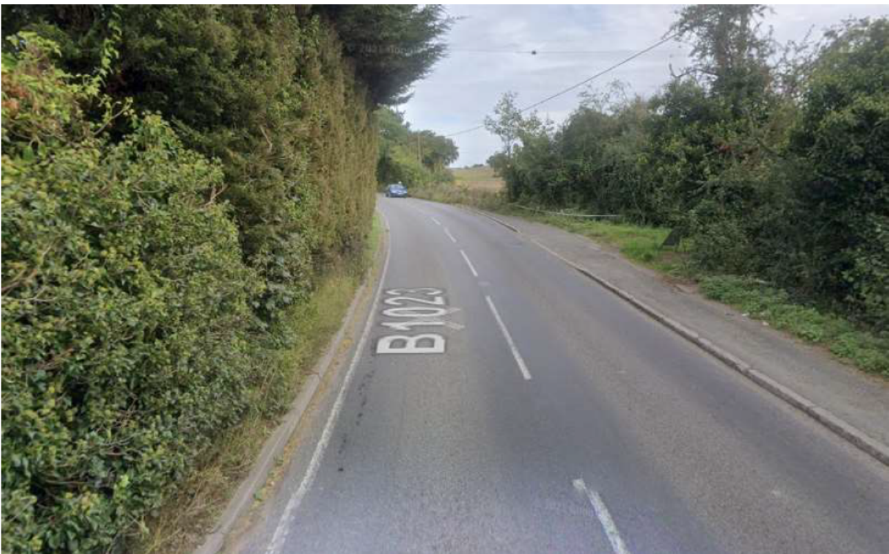
B1023 north of Inworth village (looking north) – Approximately 145m radius with no verge to allow compliant stopping sight distance
